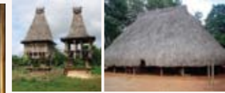
UMA LULIK thatched roof as possible wall surfaces
